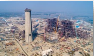
2X660 MW at Rampal, Maitree, Bangladesh-BIFPCL
